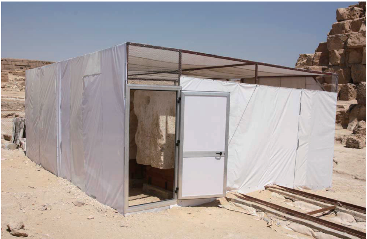
図5 鉄骨製の蓋石覆い舎 Fig.5 Steel framed shelter for the cover stones
